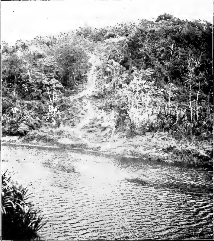
The French Location for the Bohio Dam.
