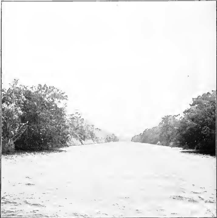
The Partially Completed Panama Canal, about eight miles from Colon.
