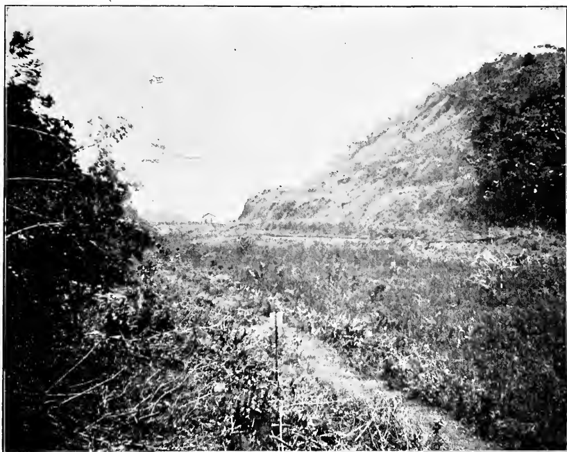
The Excavation at the Bohio Lock Site.
